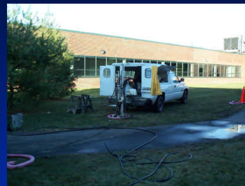
Geoprobe™ direct-push rig used to install temporary injection points
